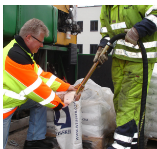
Ejector filling of bead tank
