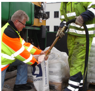
Ejector filling of bead tank
