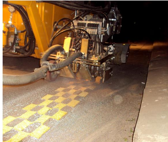
Depending on the set-up of the extruder, lines of 30 – 50 cm width can be applied. The extruder may be used for the application of various types of plain and profiled lines, single and double lines of different widths, as well as for simultaneous application of continuous and intermittent lines.
