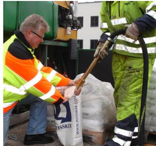
**Ejector filling of bead tank**
