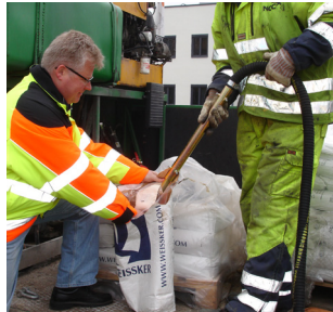
Ejector filling of bead tank
