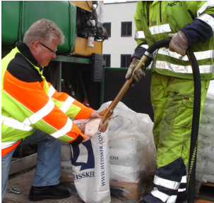
Ejector filling of bead tank
