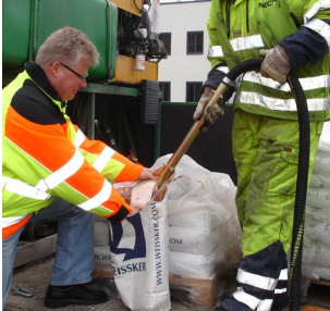
Ejector filling of bead tank
