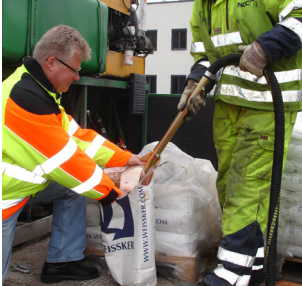
Ejector filling of bead tank
