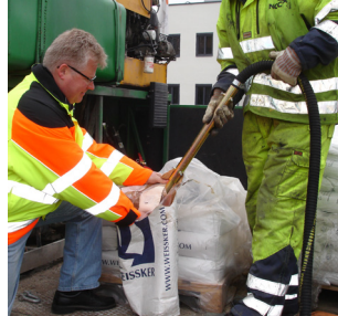
Ejector filling of bead tank
